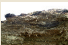
Photo IIIa. Deterioration of the upper layer
