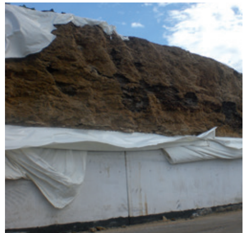
Photo 20a. Overloaded silo in an Austrian biogas plant
