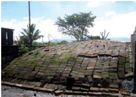
Photo 18a. Silo covered with plastics sheets and bricks in El Salvador
